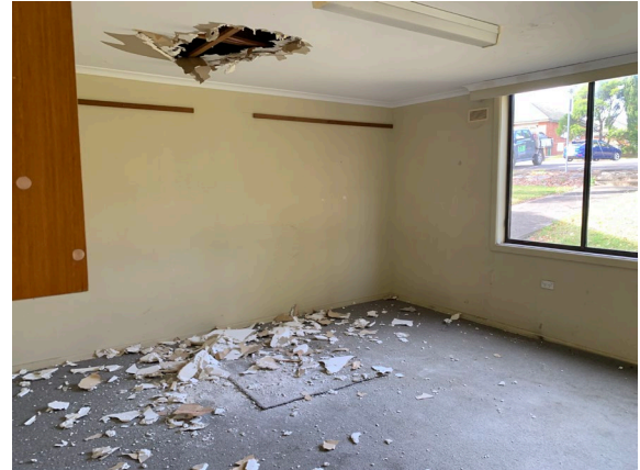
Figure 2. 20: Large hole in ceiling of bedroom in Building B1.
