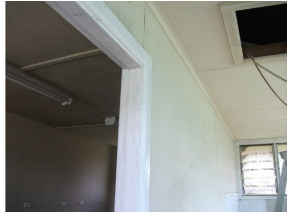
Figure 2. 18: Detail of interior of Building B4 showing internal door architrave and cornice. Source: Hazardous Building Materials Survey, Hibbs & Associates, 2014, Photograph 23, p. 59
