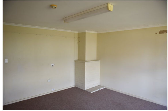
Figure 2. 14: Other half of chimney breast located in bedroom, divided by later addition partition wall.
