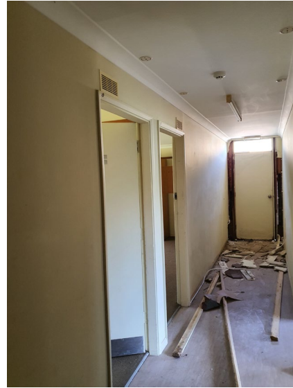
Figure 2. 10: View of bedroom door entries from central hallway. Note removed architraves to fire exit door and scattered debris.
