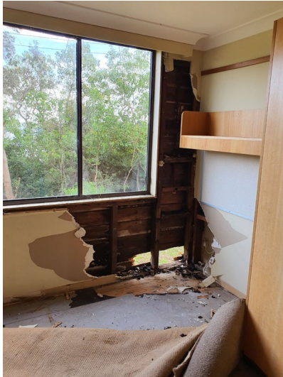
Figure 2. 19: Internal wall lings removed revealing internal timber structure and missing external weatherboards to Building B3.
