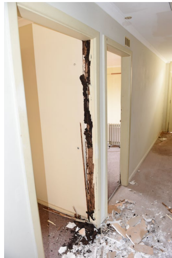
Figure 2. 22: Evidence of termite damage to architrave in Building B1.
