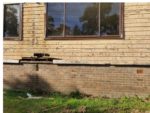
Figure 2. 25: Peeling paint and missing and damaged weatherboard cladding to Building B3.
